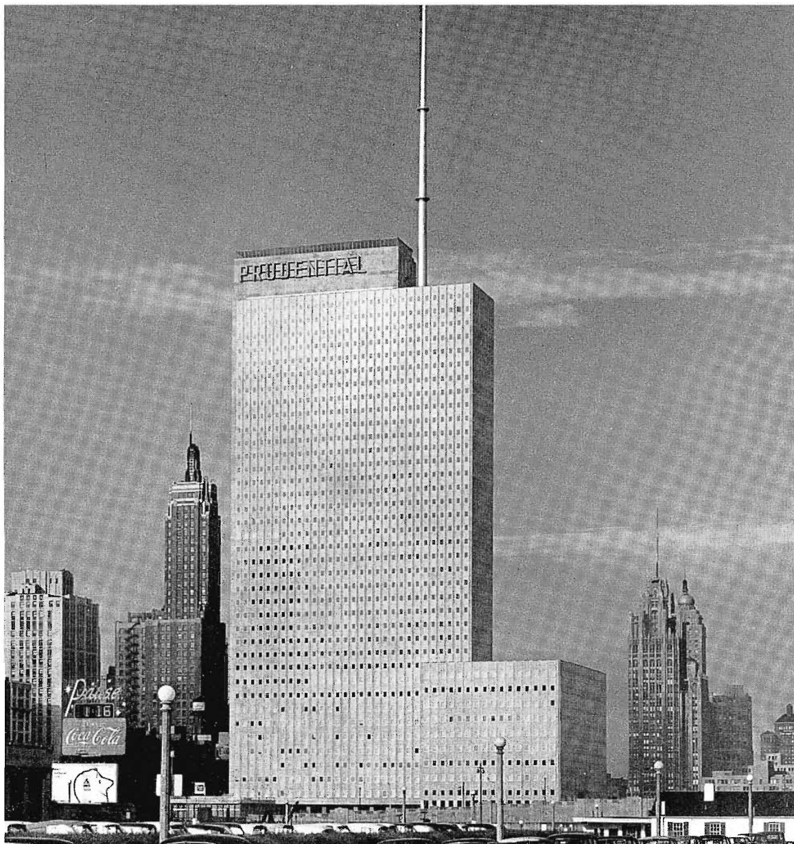
FIG. 1. Located atop the Prudential skyscraper, WGN's unique tubular steel tower is Chicago's newest landmark.
