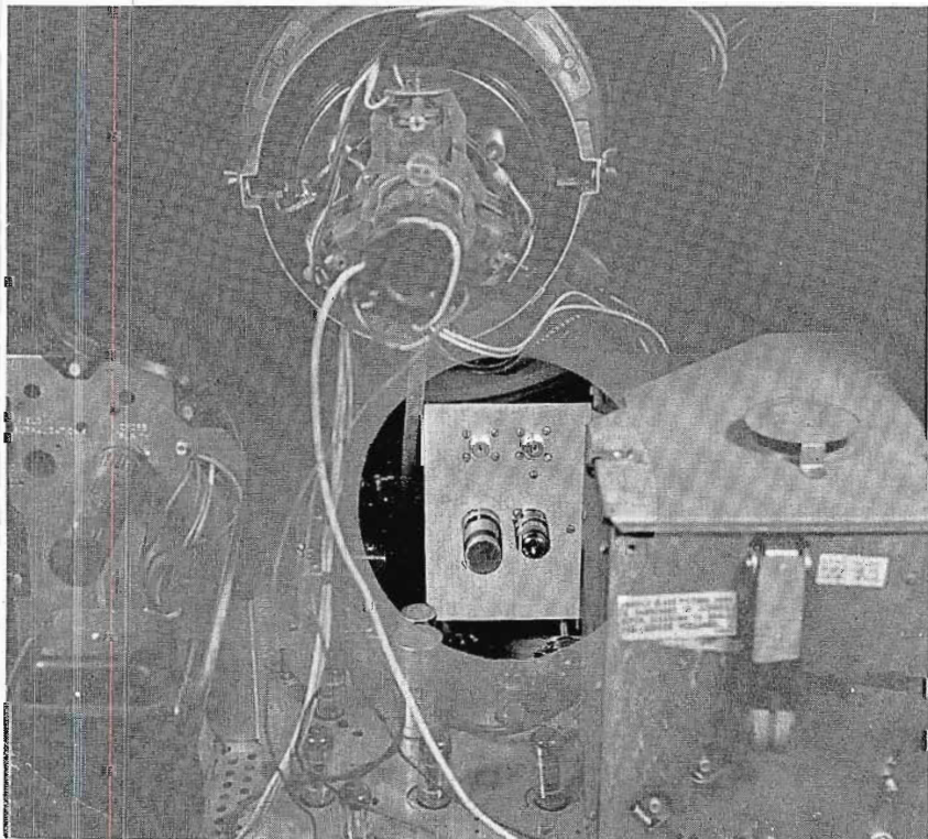
FIG. 4. The preamplifier is shown mounted in the 21CT-55 color TV receiver.
